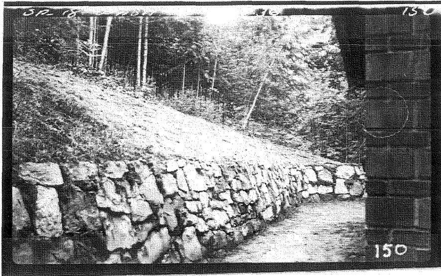
TSP11: Stone retaining wall behind superintendent's house. Unknown photographer. 1936
