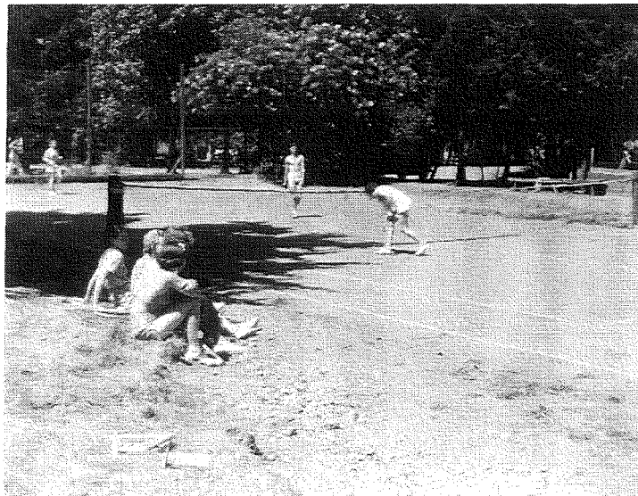
TSP12: Tennis courts. Dan Sheehan, photographer. July, 1936
