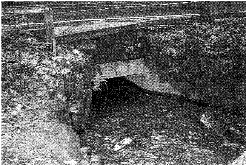
0028: Highway culvert, north elevation, looking southwest.
