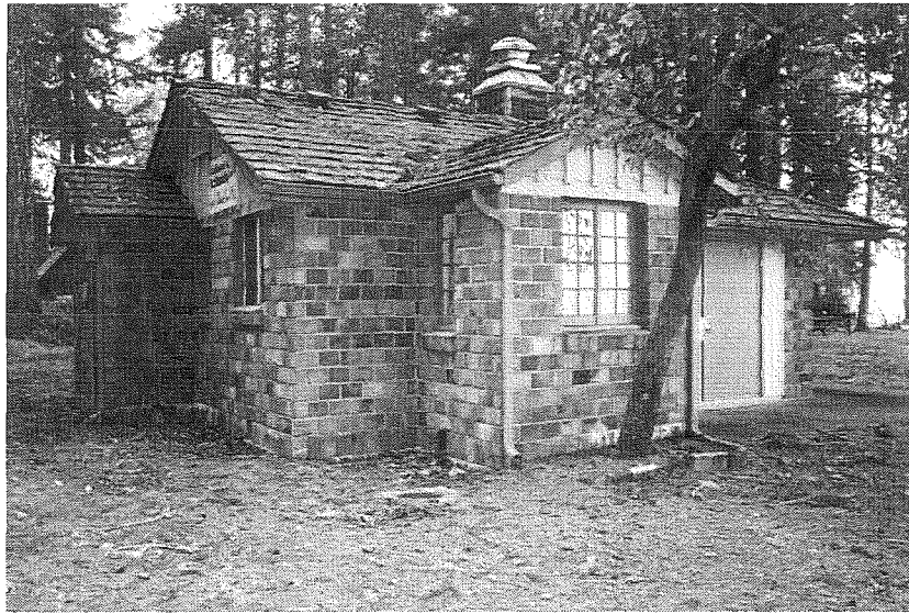
0019: Building 16 (concession), south and east elevations, looking northwest.
