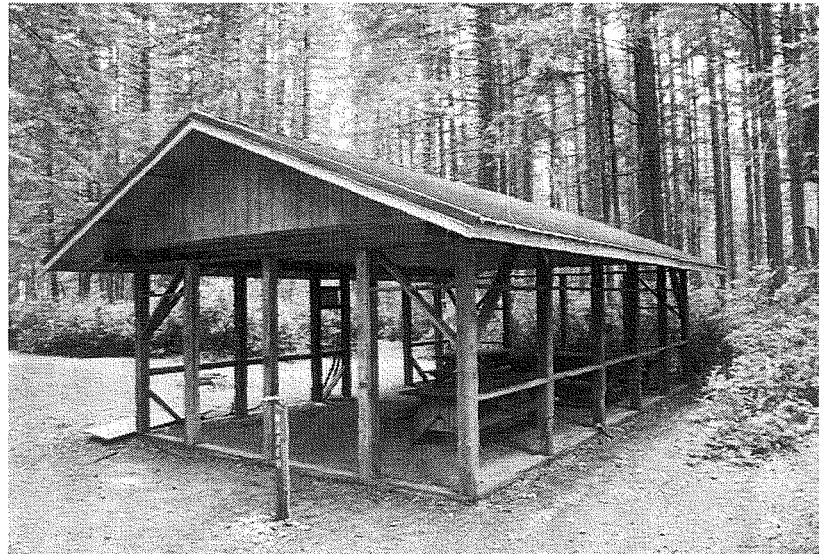
0046: Building 20 (group camp shelter), north and west elevations, looking southeast.
