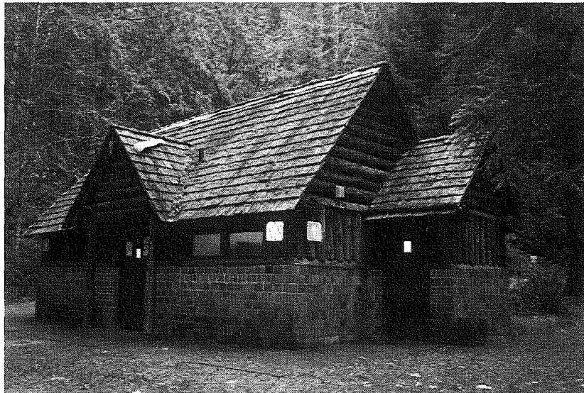
0034: Building 8 (comfort station #3), north and west elevations, looking southeast.
