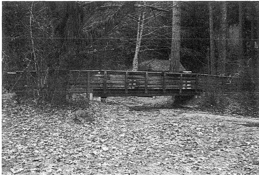
0005: Lower footbridge, north elevation, looking southwest.
