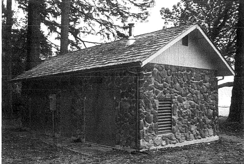
0003: Pump house, northeast and southeast elevations, looking west.
