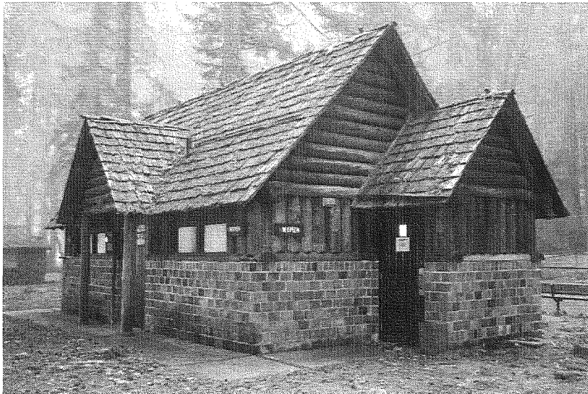
0016: Building 6 (comfort station #1), north and west elevations, looking southeast.
