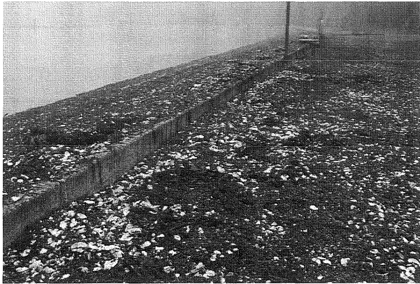
0017: Seawall, looking east.
