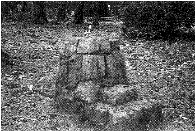
0004: Typical drinking fountain, looking northeast.
