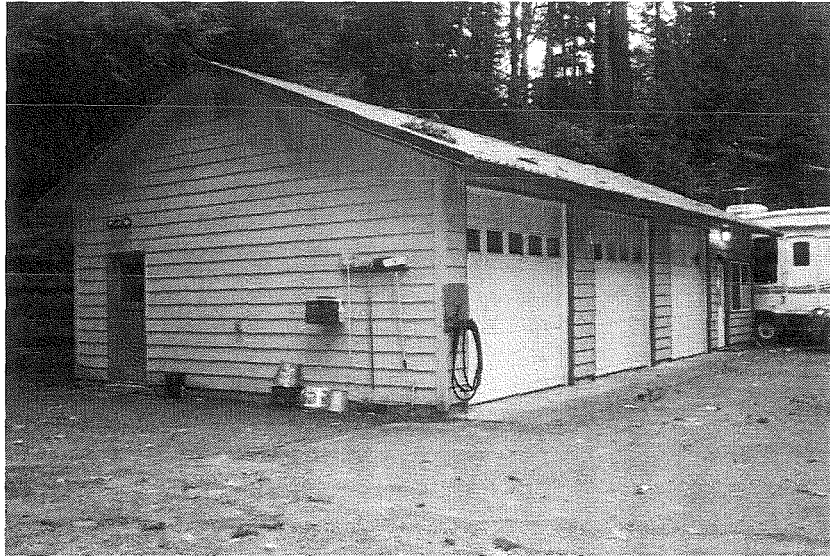
0043: Building 25 (modern office/garage), north and east elevations, looking southwest.
