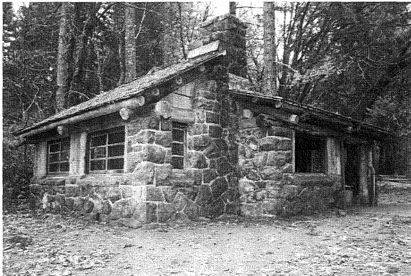
0006: Building 11 (shelter kitchen), northwest and northeast elevations, looking south.
