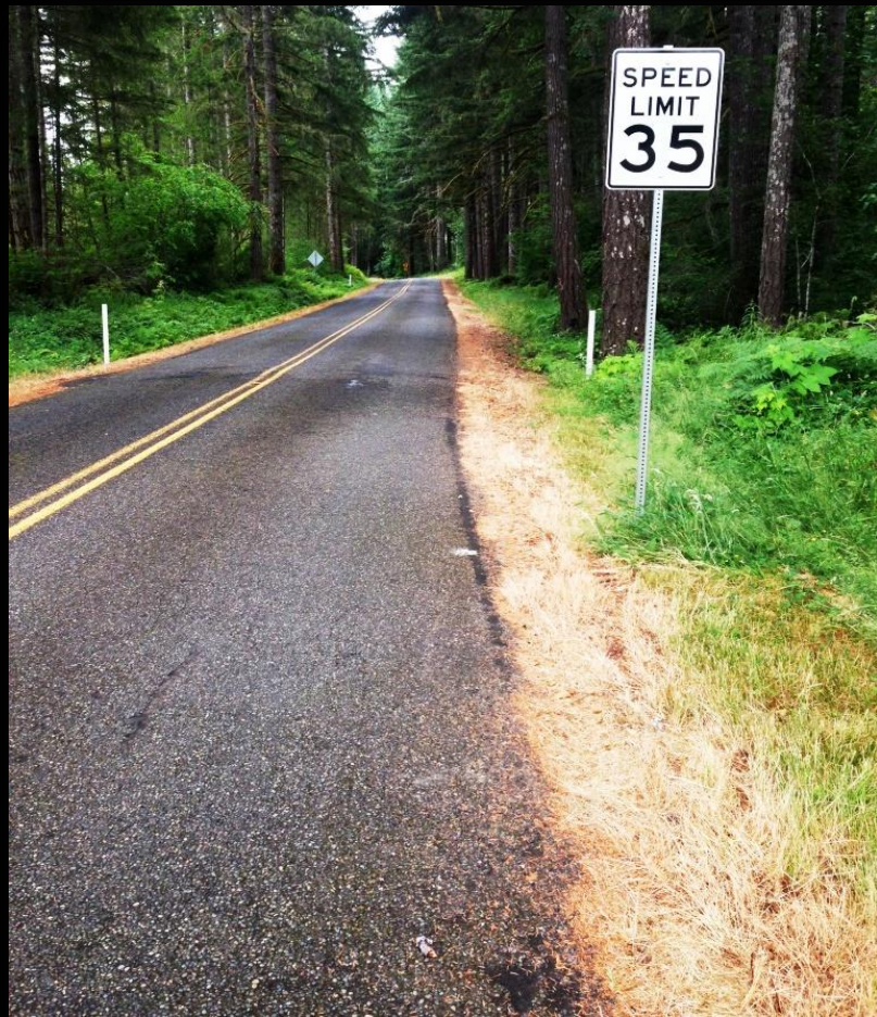
Chip Seal Elfendahl Pass Belfair
