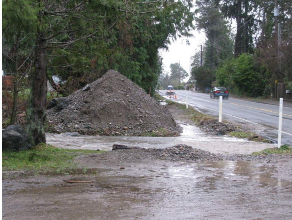
Twanoh Falls Creek – December 13, 2010 - monitoring/flooding event
