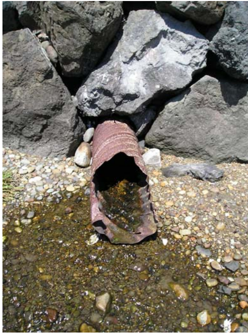
Small drainage along the Northshore of Hood Canal
