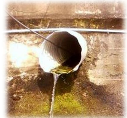
Photo 26 Culvert Monitoring Location
