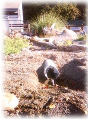
Photo 36 Culvert Monitoring Location
