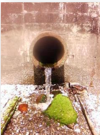
Photo 23 Culvert Monitoring Location
