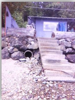
Photo 33 Culvert Monitoring Location
