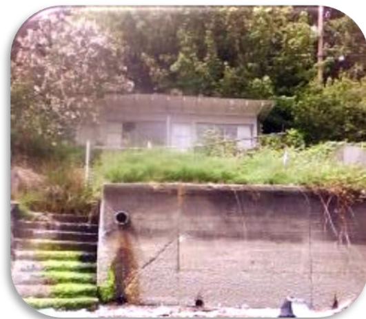
Photo 41 Culvert and Stair Seep Monitoring Locations
