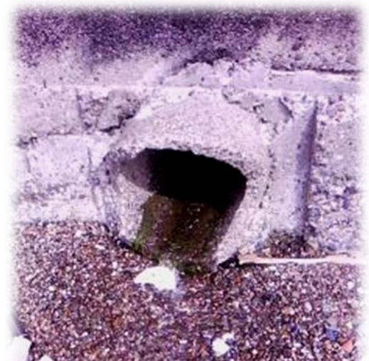
Photo 16 Culvert Monitoring Location
