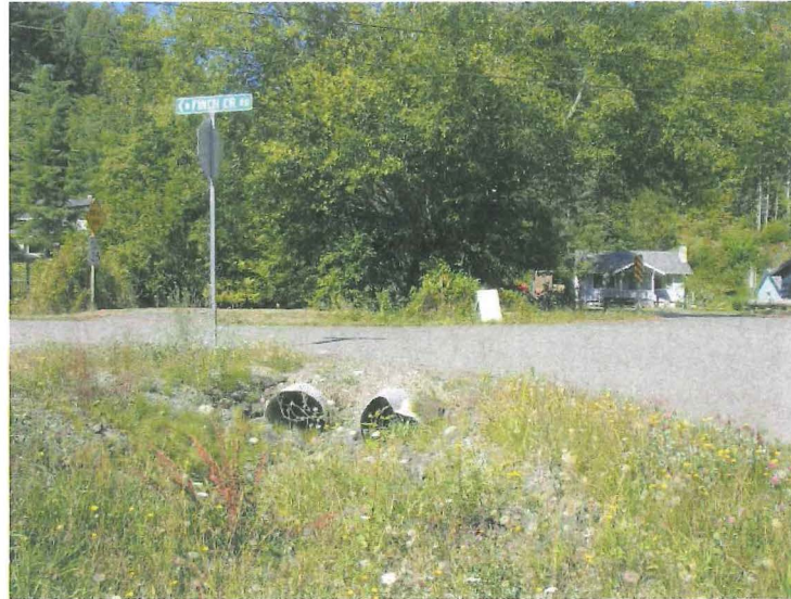
Culverts at SR 119
