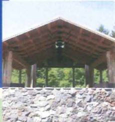
Environmental Learning Shelter-Orientation Kiosk under canopy
