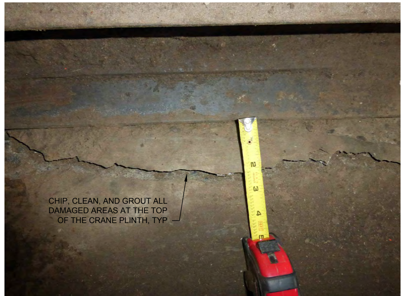
TOP OF PLINTH REPAIR DETAIL N.T.S.
